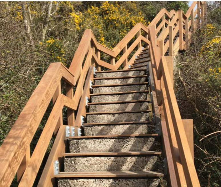
Wooden Handrail Installed
