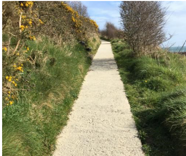
Upper Path Car Park Access - Grip Surface
