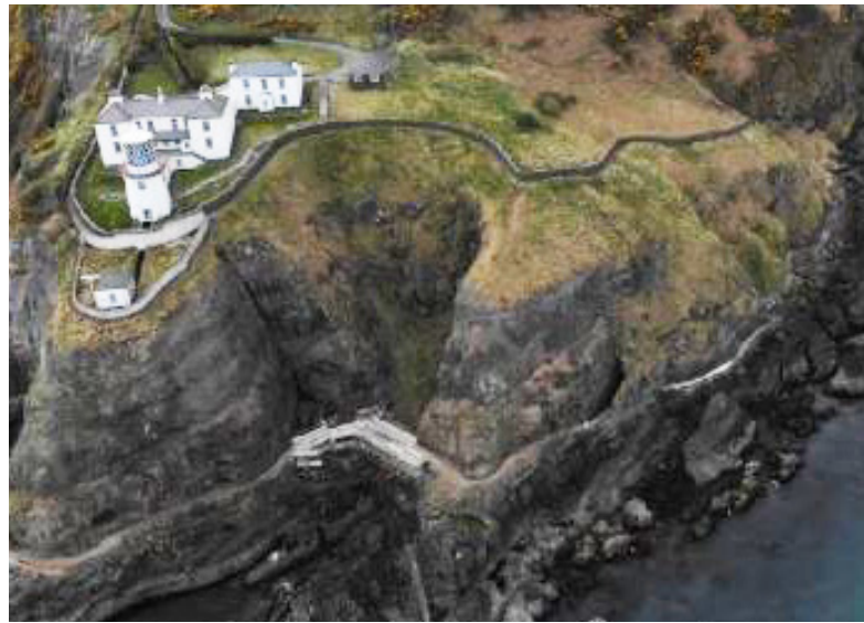
Section B Bridge Works And Path Repairs
