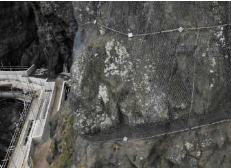
Netting Installed On Cliffs
