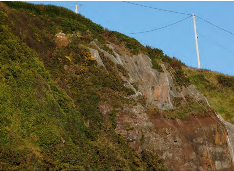
Descaling and vegetation clearance on the cliff face
