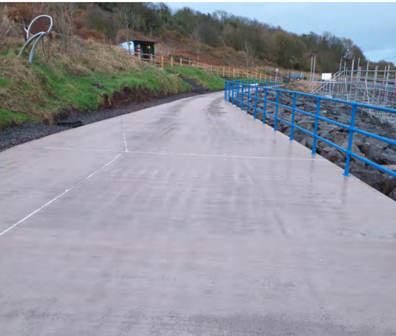
New handrail being installed along the promenade
