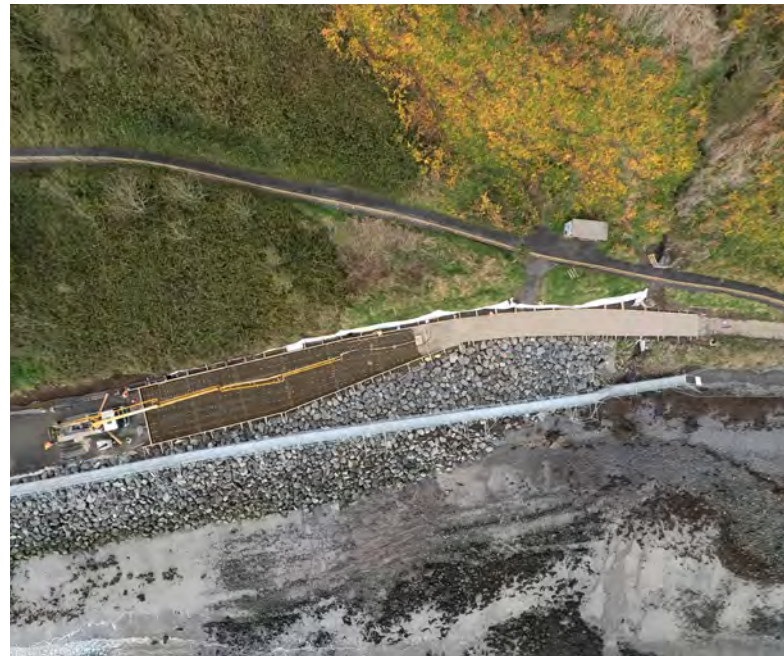
Pouring the next section of the promenade
