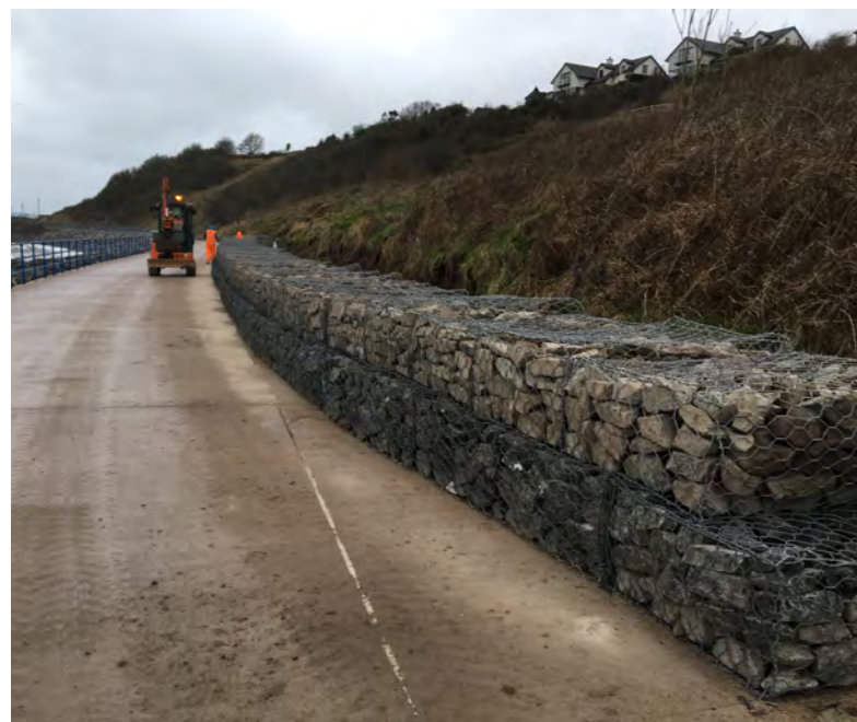
Gabion basket continues to be built and filled along the promenade
