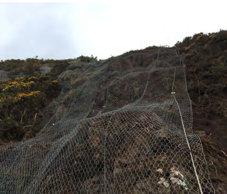
First of the new rock fall netting installation completed
