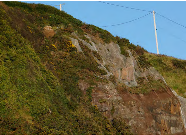
Cliff face after scaling and prior to netting installation
