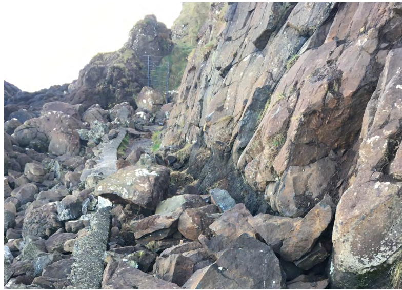
Debris after heavy scaling has been completed
