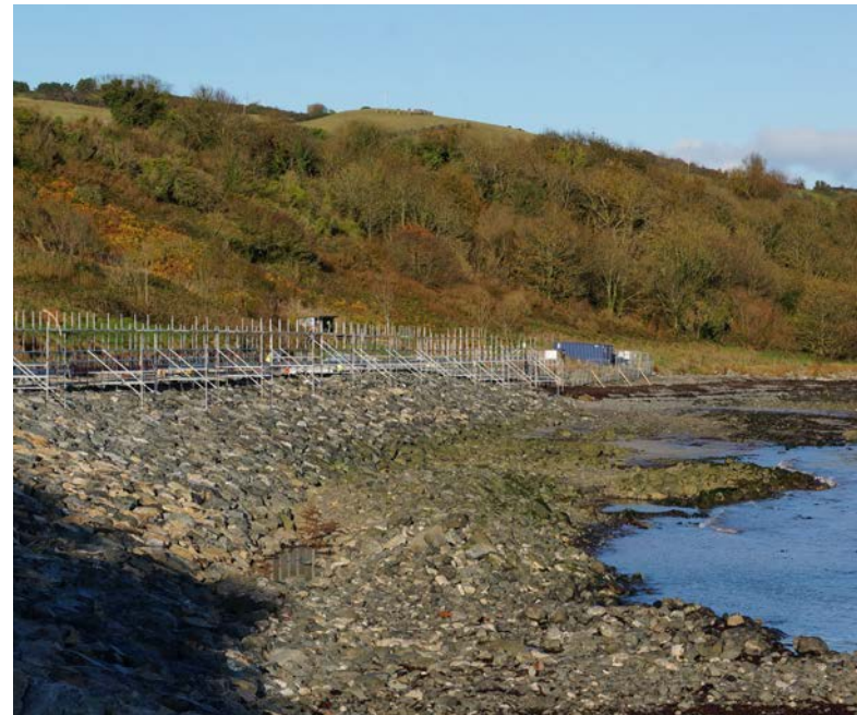
View north of the rock armour revetment
