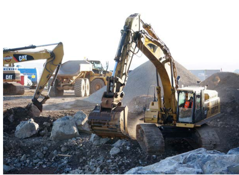
Last section of rock armour revetment underway
