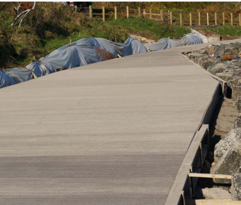
New promenade surface of reinforced concrete with brush finish
