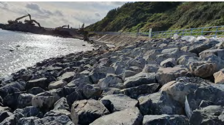
Rock armour revetment works viewing South
