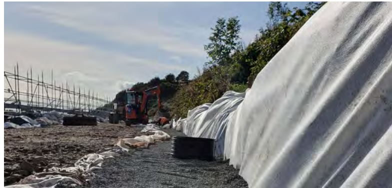
New promenade drainage installed at the toe of the bank
