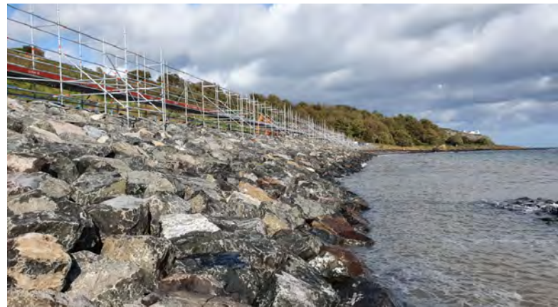
Temporary scaffold walkway for site operatives
