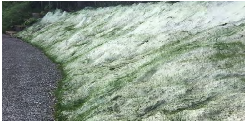
Grass coming up on the pre-seeded erosion mat covered bank
