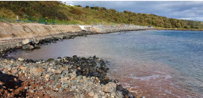
Rock armour revetment works view North
